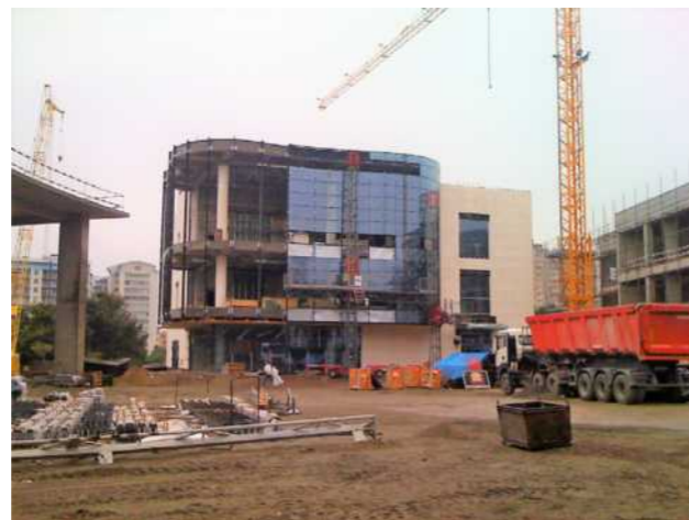
Construction of ADA Library
